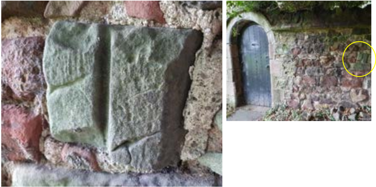
Figure 16- This piece of stonework had been added to the west wall of the precinct. It appears to contain a slot for a pane of glass and distinct carvings on the window frame.
