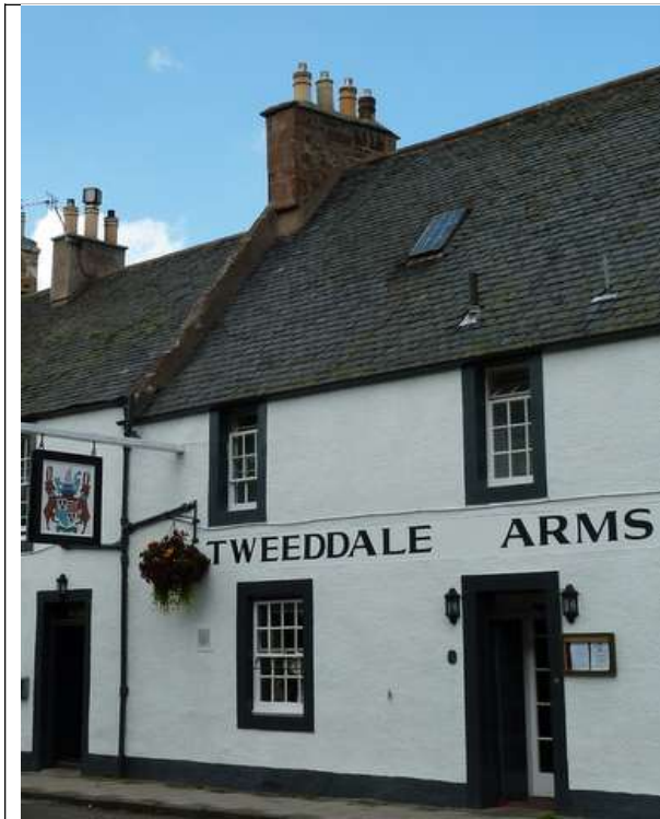
Fig 4 Note the thackstone at the base of the chimney stack and stone riggings.
