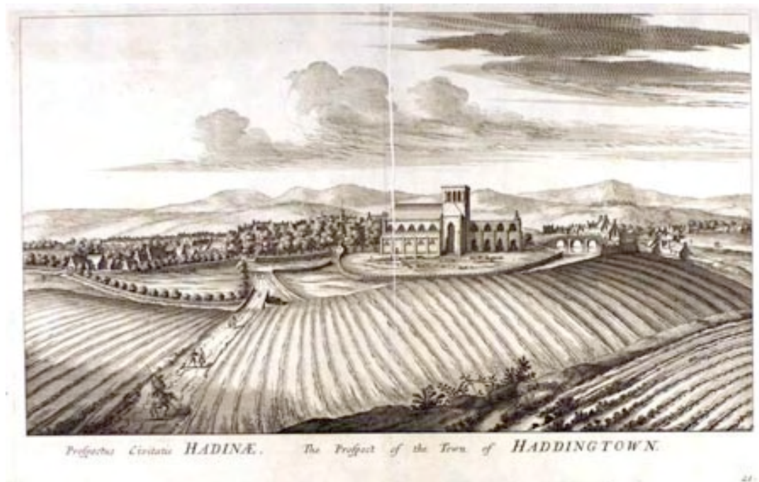
Fig 3.11 – Sleazar’s engraving of Haddington dated 1693 depicts the vista from Monkkrigg. The burgh wall, Poldrate Bridge, Nungate Bridge and the battered St Mary’s are all recognisable features.
